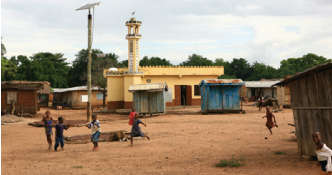
Wilkin Solar, an E+Co borrower that sells solar systems and lanterns throughout Ghana, installed four solar-powered street lights in the town of Jama, Ghana.
